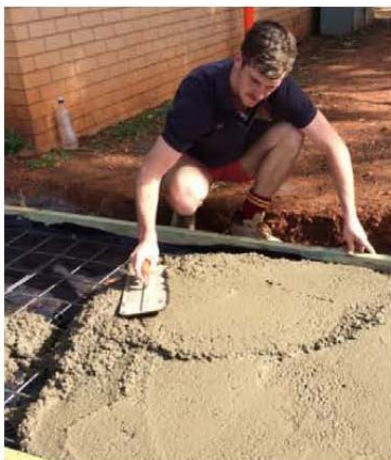
Left: Chad Hartin floating a concrete slab (Peak Hill)
